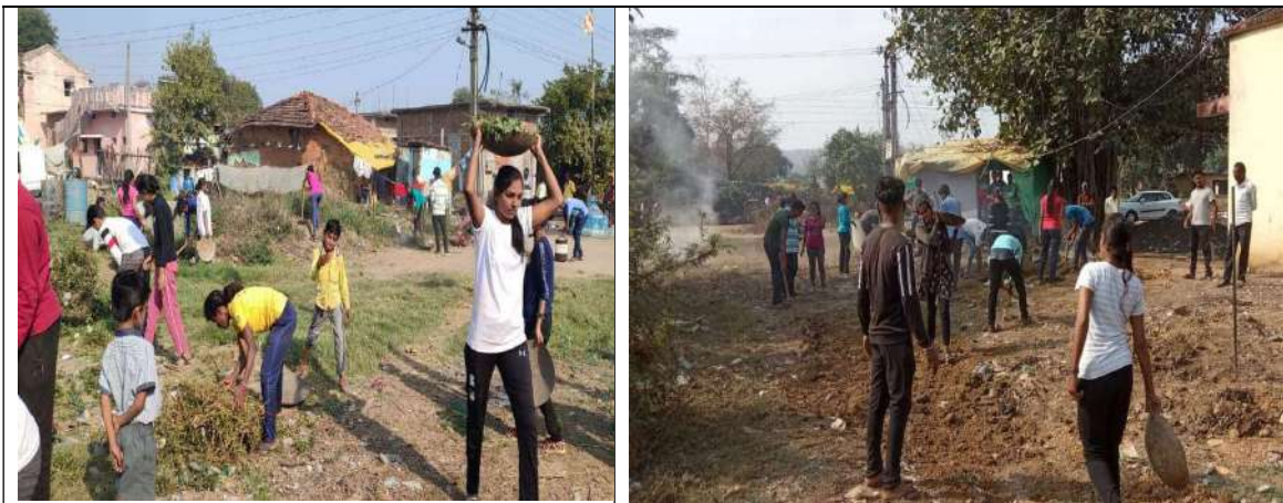
The campers constructed a 300 metres double bypass road
